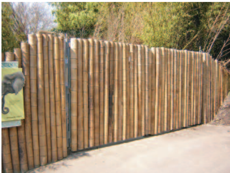
Photo 2. Fence of bamboo poles in the Rotterdam zoo in the Netherlands. Photo P. van der Lugt.
